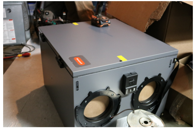
Honeywell TrueFRESH HRV during installation
